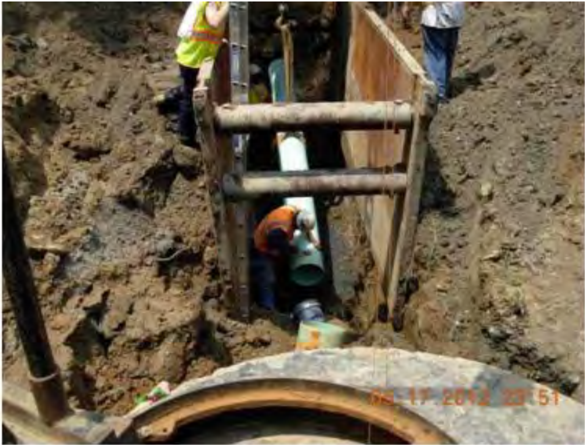
Figure 9: Typical Gravity Sewer Construction
