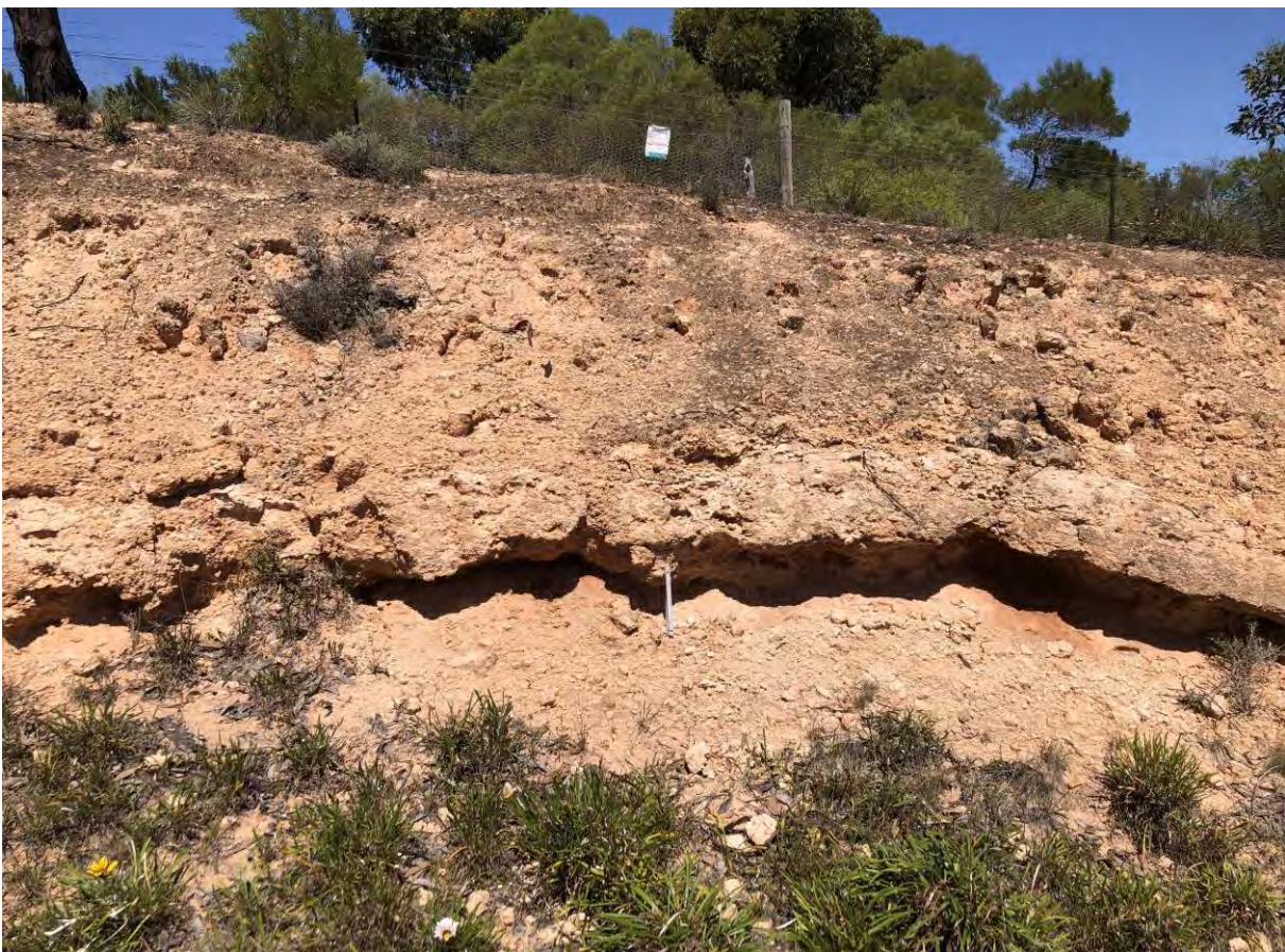
Figure 5: Extremely Weathered Calcrete on a Cut Batter (near BH12, Facing Northwest)
